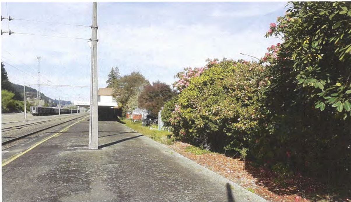
OPTION C looking east. The dock platform track is still in place under the leaf litter.
