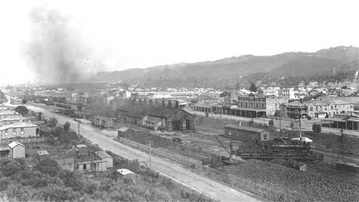
Taumarunui circa 1923 showing the smoky hazy that emanated from every engine shed in the age of steam. An X-class is being turned on the turntable, something that normally had to done after each trip because they primarily worked trains over the central section of the NIMT to Taihape.
