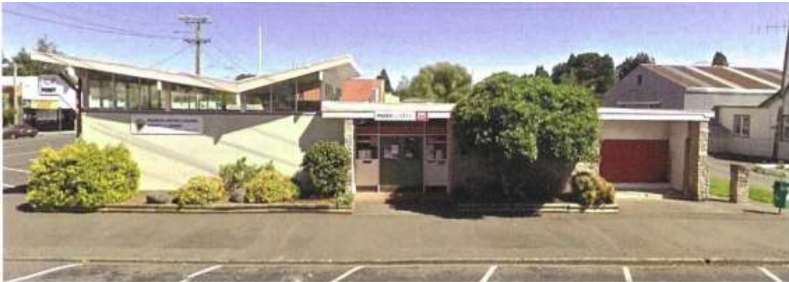
Figure 4.3: Street view of Raetihi Service Centre from Duncan Street
