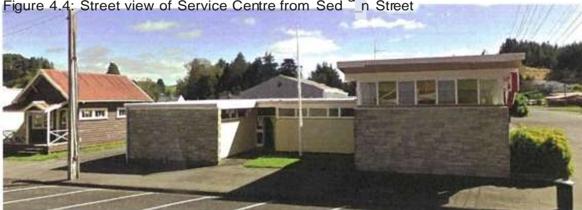
Figure 4.4: Street view of Service Centre from Seddon Street
