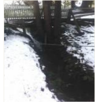
Choke in Miro Street watercourse - tributary in Ohakune
