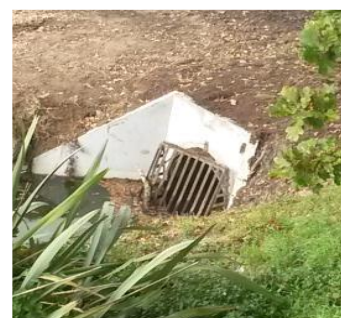
Installing a New Wing Wall, Taumarunui
