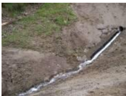
Improving Outfall of Stormwater
