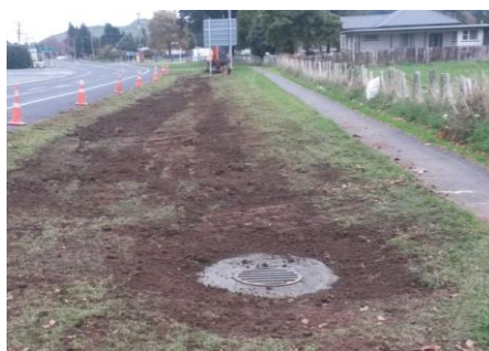
State Highway 4, Raetihi New Stormwater Line
