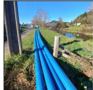
Figure 5 New watermain pipes
