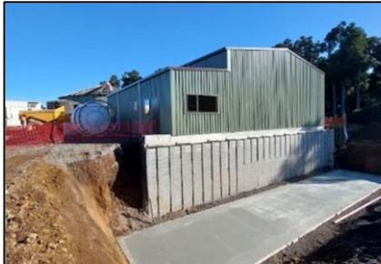
Figure 4 Progress at Ohakune Water Treatment Plant
