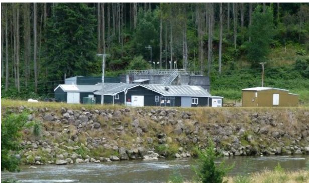
Figure 20 Water treatment plant examples in Taumarunui
