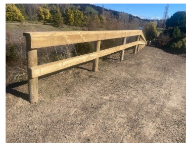
Taumarunui River walkway fencing
