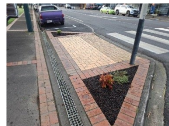
Taumarunui Garden renovations
