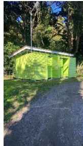
Taumarunui Riverside Toilets refurbishment
