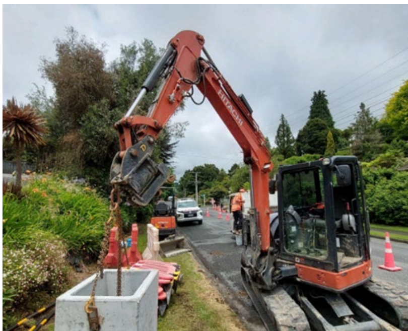
Stormwater Pipe and Catchment Pit works
