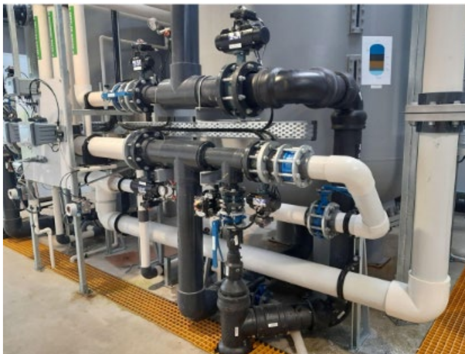
Newly installed Check Valves and Pipework re-arrangement
