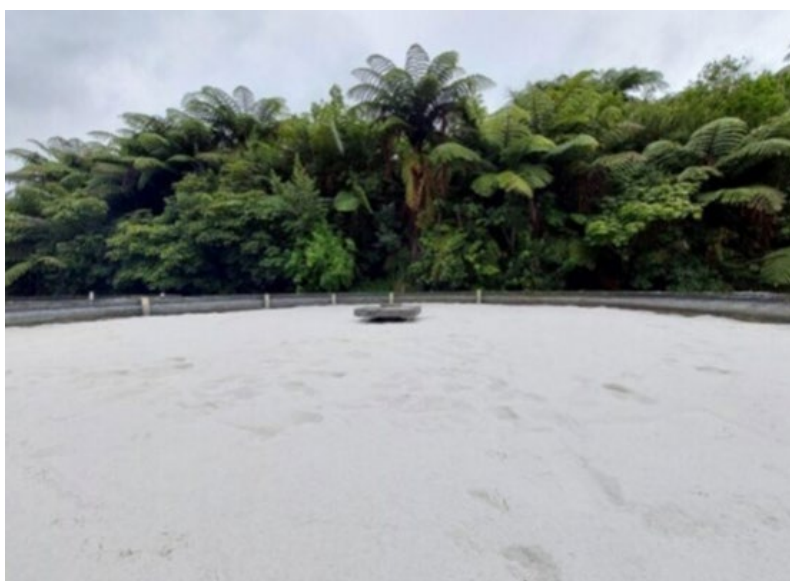
New Sand Media in Sand Filter No.2 at Pipiriki WWTP
