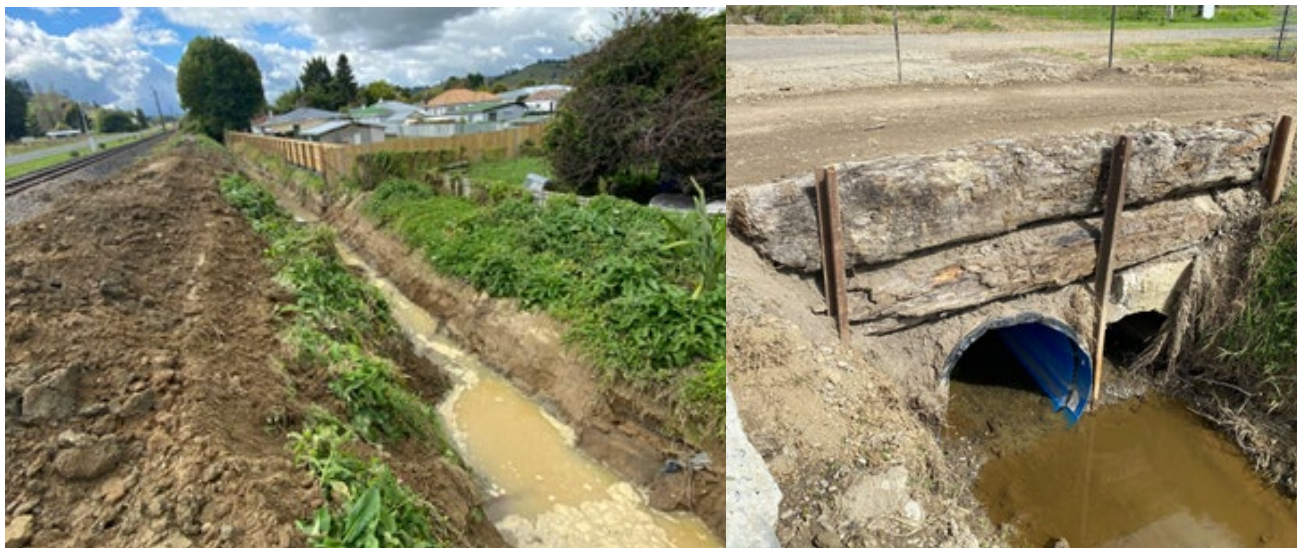
Mitigation works along the Totara Crescent Railway Corridor
