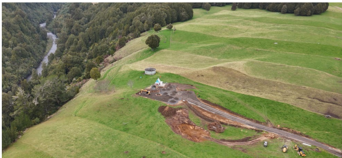
Ōwhango WTP Access Track works
