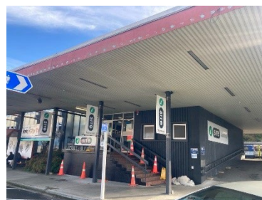
Taumarunui I-site upgrades
