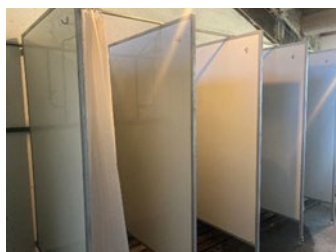
Shower Facilities, Taumarunui Jubilee Grandstand- Men's
