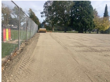
Christie Park Volleyball Court Renovations
