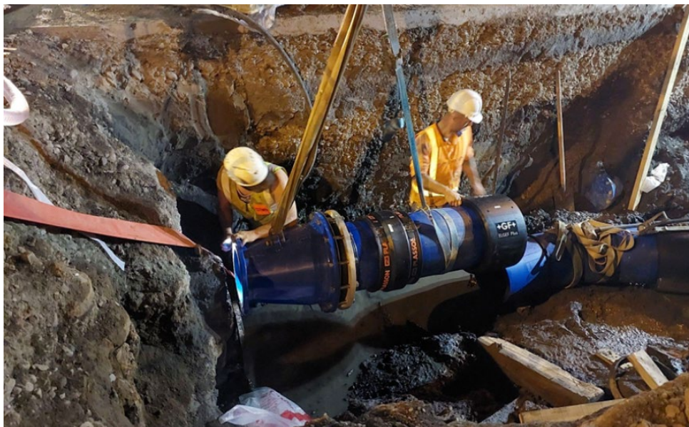
Hakiaha Street watermain installation works
