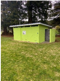
Taumarunui Esplanade toilets refurbishment
