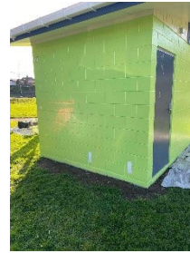
Taumarunui Domain Toilets refurbishment
