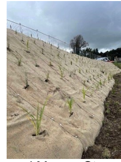
Taumarunui Morero Stream project
