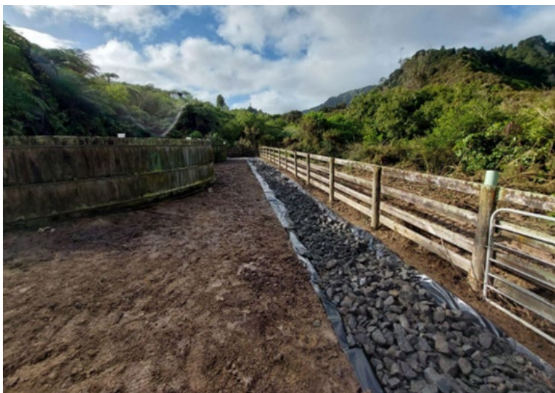
Access Improvement works at Pipiriki WWTP
